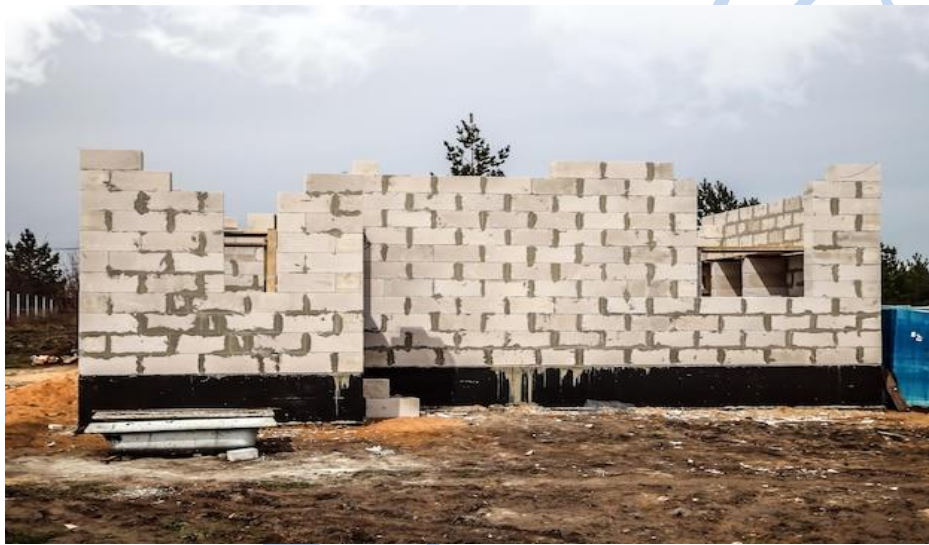
Figure 1. Processes of their construction from aerated concrete building bricks
